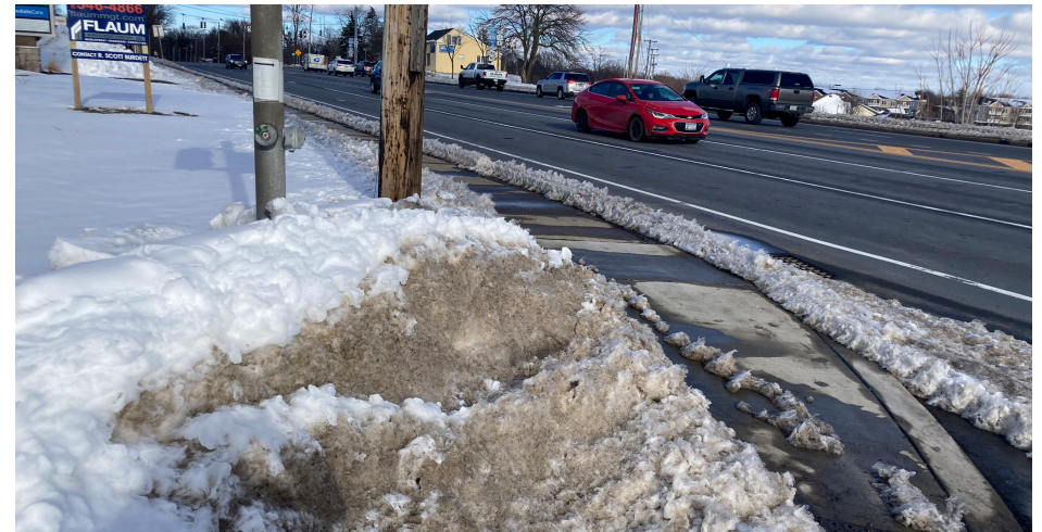
Snow pile blocks access to pedestrian push button and curb ramp (Chili Avenue).
