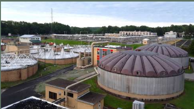
Monroe County Water Resource Recovery Facility
